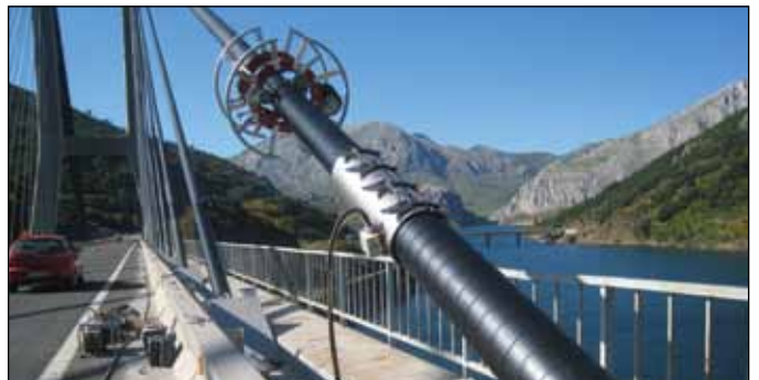
2. Using an electric heating blanket, heat the wrap for 5-10 minutes to create a permanent bond.
