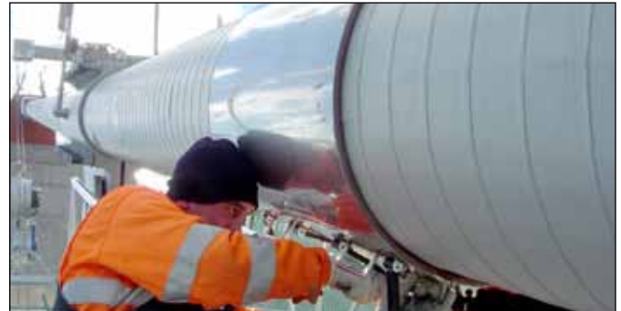
2. Using an electric heating blanket, heat the wrap for 5-10 minutes to create a permanent bond.
